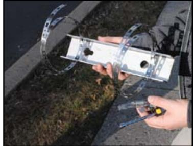
**Step #2** - For the most accurate results, the bracket should be installed so the Radar Recorder is facing traffic on a 45 degree angle. Once you have determined this position, wrap the bands around the pole and place the bracket.
